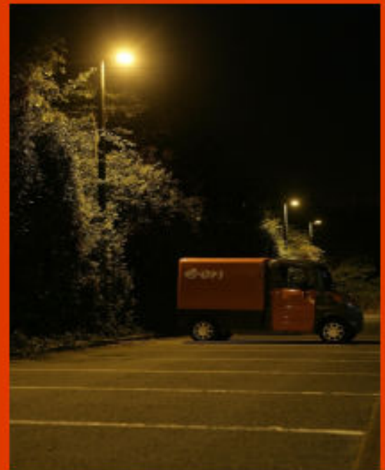
Before – 70W Son Installation 90 circuit Watts per lantern
